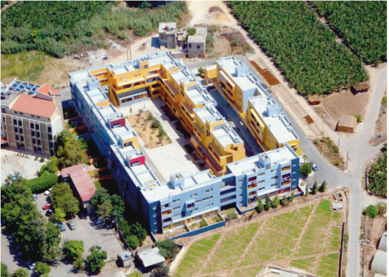
Above: Aerial view of the project. Photo by Joumana Jamhuri
